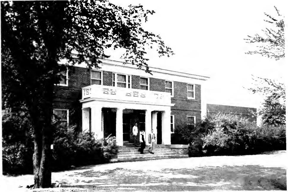
Entrance to the new Infirmary
